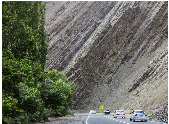
Figure 3: Chalus Road, Northern Iran
